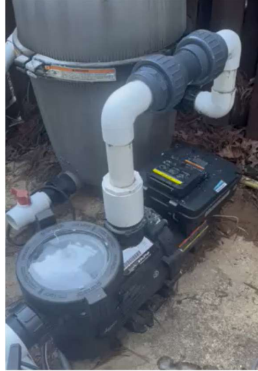
Shaft on swimming pool
